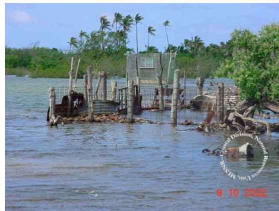
Plate 4.6: (above) Abandoned house and flooded pig fence at Kanokupolu. Water height is approximately 1-2ft deep
