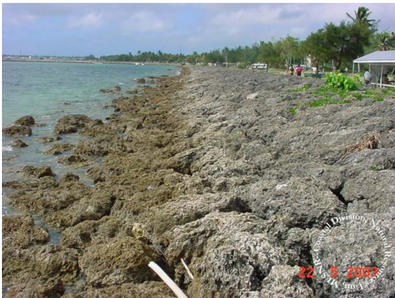
Plate 5.1. The Coastal Protection Wall at Nuku'alofa Waterfront
