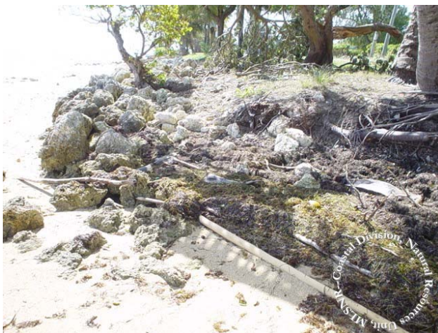
Plate 4.9: The seawalls at Manuka, where it has been breached by recent tidal waves, exposing coastal tree roots and ultimately brought it down at places. (Picture taken in early 2003)
